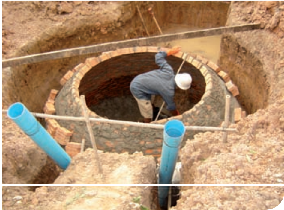
Domestic biogas digester under construction. SNV Cambodia.
